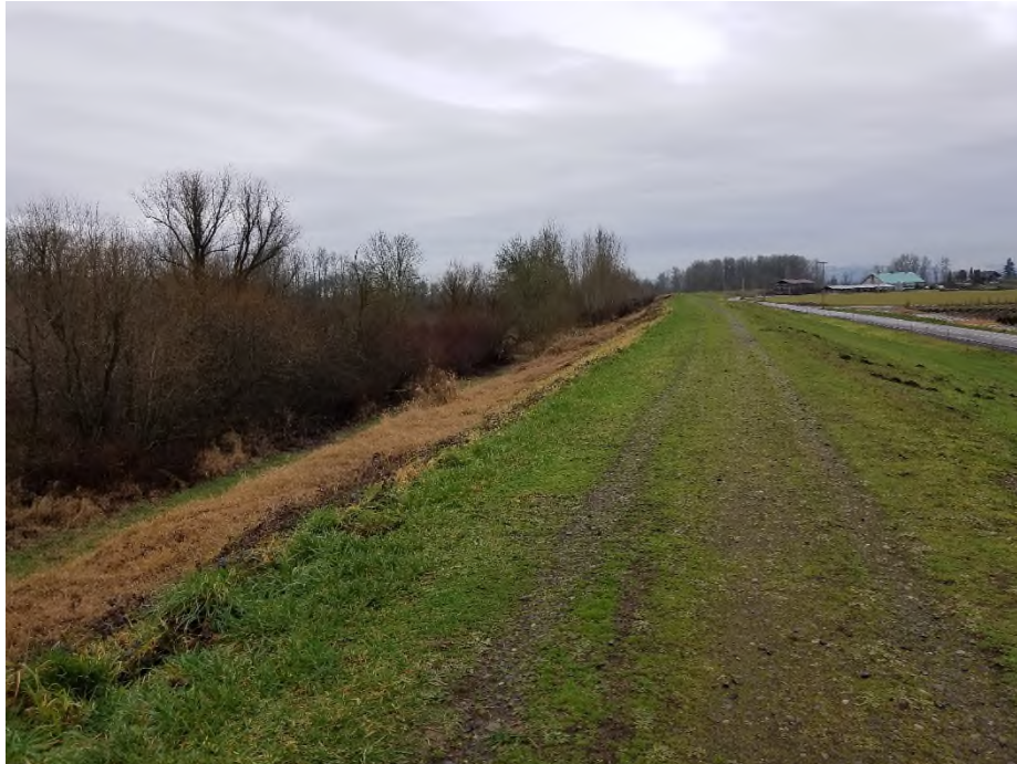
Southern Floodway portion of Chapman Landing - view from the Dike
